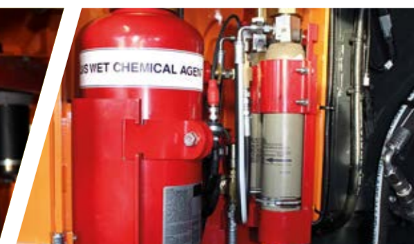
Automatic fire suppression system
