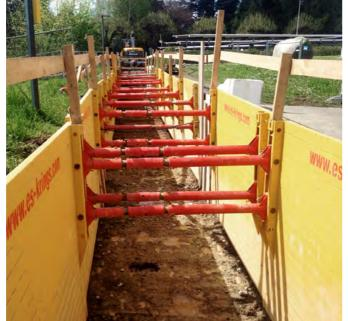
The little KVL steel box is ideal for inner-city areas, the sturdy KS 60 is recommended for inner-city sewer construction projects, and the KS 100 is designed for use at greater depths.
