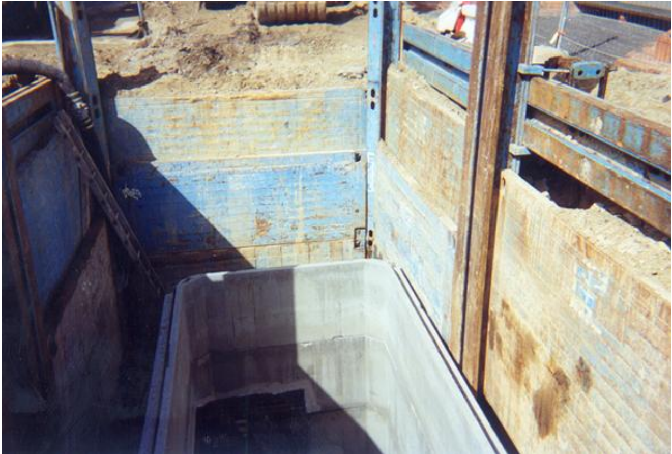
↑ Double slide rail for corner post
